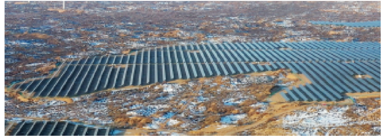
Ground-mounted power station project in Shan Xi Province, China
