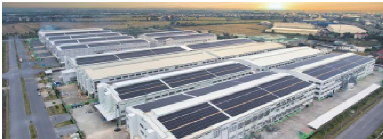
Distributed Project in Vietnam
