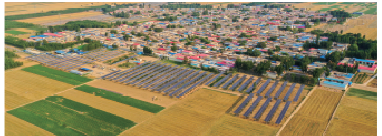
Tracker power station in Hebei Province
